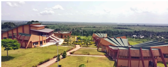
Classrooms (at right) & auditorium (at left) of the IMPS
